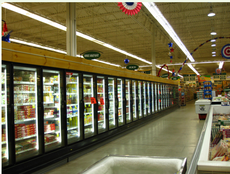
Fresh County Market, a Self-Help borrower in Gary, Indiana, installed LED lighting in their refrigerated cases.
